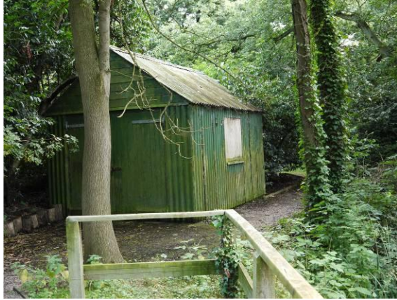
Pump house of 1946
