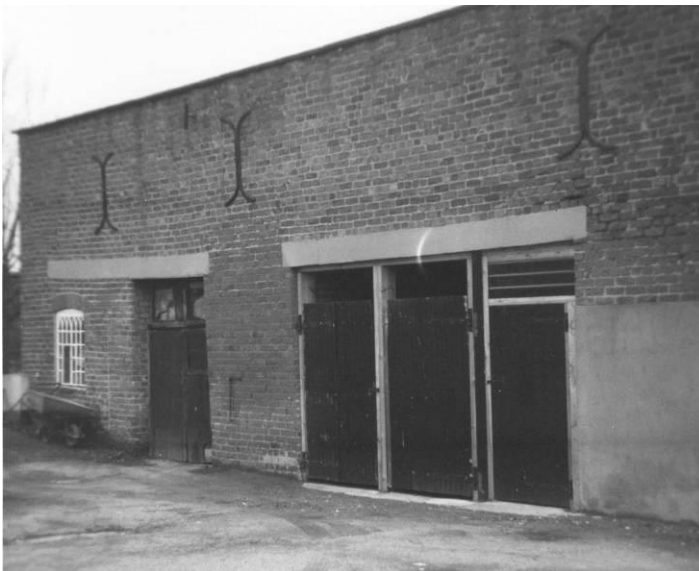
Undated photograph of 18th c (?) building shown on Tithe Map c1842. Note cast iron window frame. (Box of information collected by Des Carroll)
