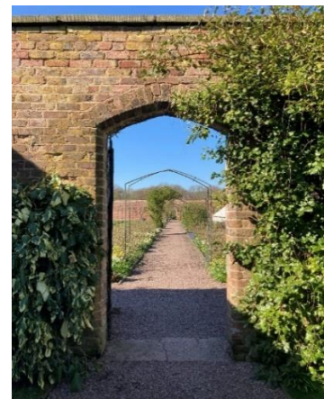
Eastern Entrance with pointed arch
