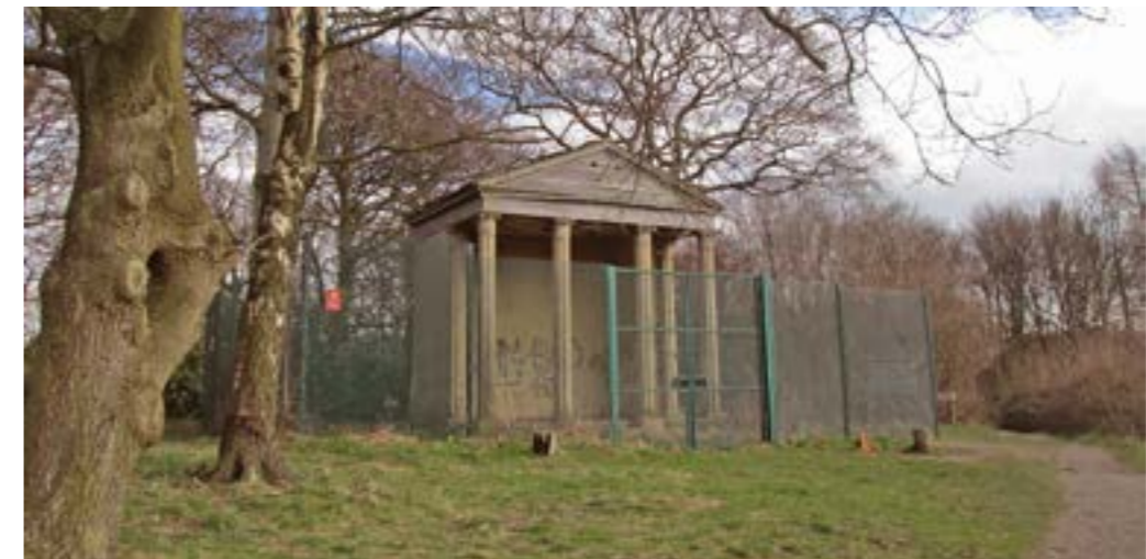
Derelict Little Temple, Temple Newsam, 2015 (Upgraded to Grade II* 2016). © Sarah Rutherford.
